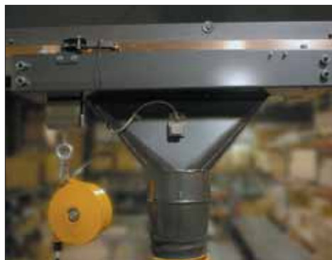
Monoxivent's Exhausting Rail/Trolley - exhausts toxic fumes through the plenum and to the main duct system. The trolley features a pressure switch, roller contactor, and stabilizing wheels/rollers.
