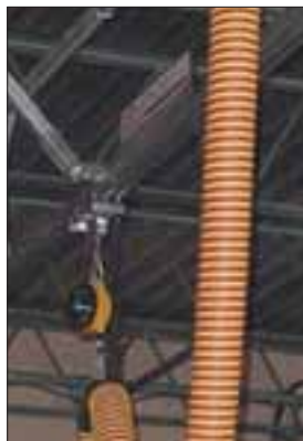
Track/Balancer/Hose Assembly - shown on the AXPT system.
