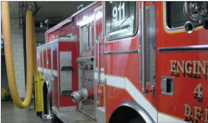
The AXPT installed system, with high visibility red/yellow hose assembly and signature Monoxivent Safety Boot.
